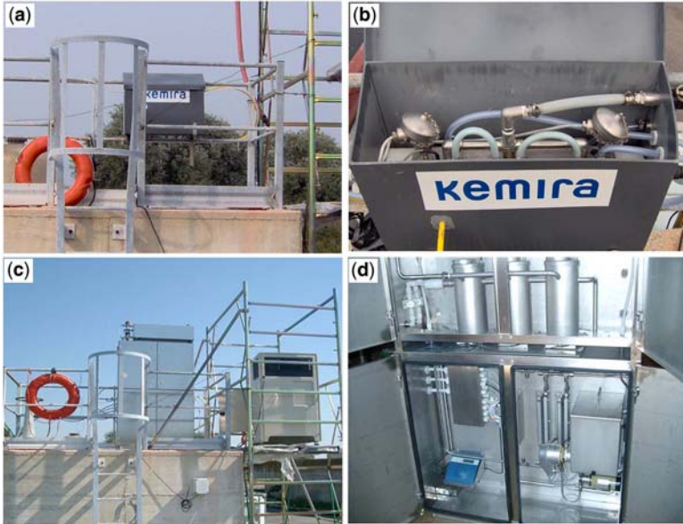
Figure 54 The first PFA hydroform production system (kemira Oyj) used in full-scale studies: prototype (a, b – 2005) and pilot system (c, d – 2006).
